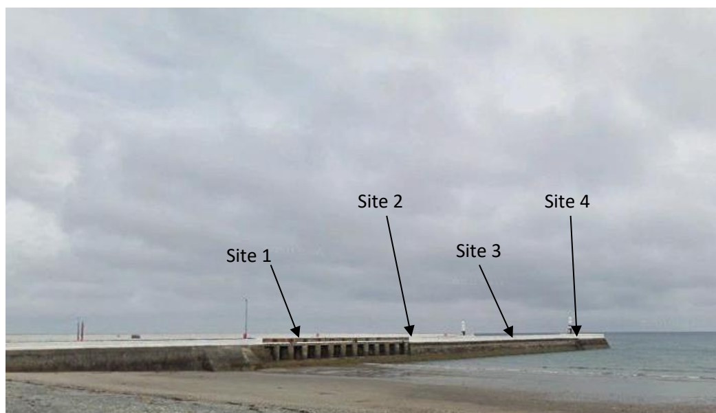
Figure 1. Positions of the four survey points along the southern wall.
